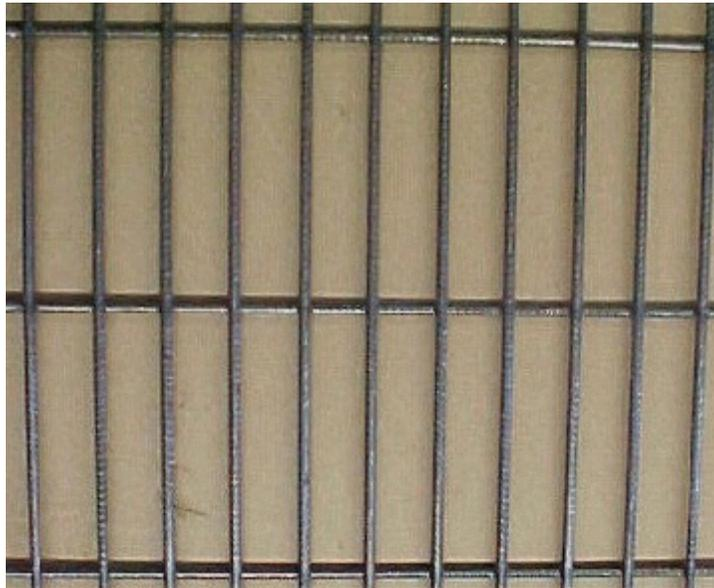
For deformed steel wire, deformations should be spaced along the wire at a uniform distance and should be symmetrical around the perimeter of the section. The deformed wire should have two or more lines of deformations. The average longitudinal spacing of deformations should be 3.5 to 5.5 deformations per inch in each line of deformation on the wire.
